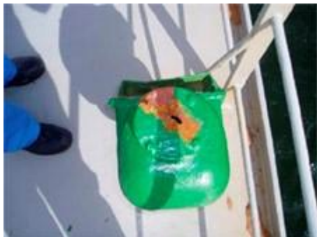
Ballast tank vent on the deck of a ship has a hole.
