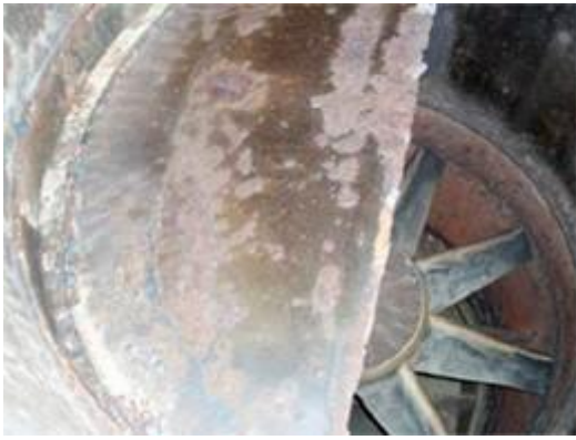
Fire damper stuck in closed position and it has been cut in half to let air escape.
